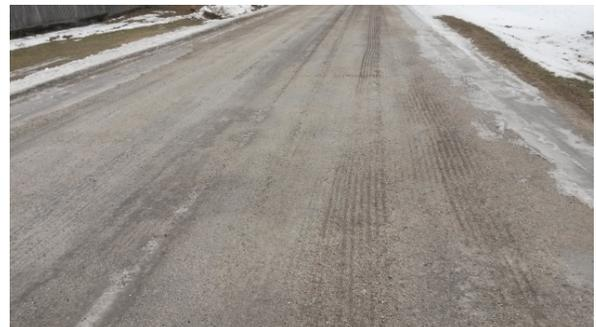
the seal coat, it is possible that furrows may occur in the seal coat after this process takes place.
