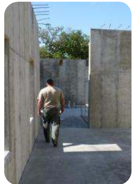
Community safe room under construction
